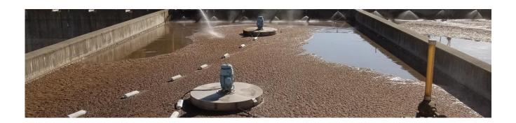
The activated sludge process utilizes aeration and biological floc composed of microorganisms to treat sanitary and industrial wastewater. This process is applied in a wide variety of systems including conventional activated sludge treatment plants, oxidation ditches, sequencing batch reactors, and package plants.
